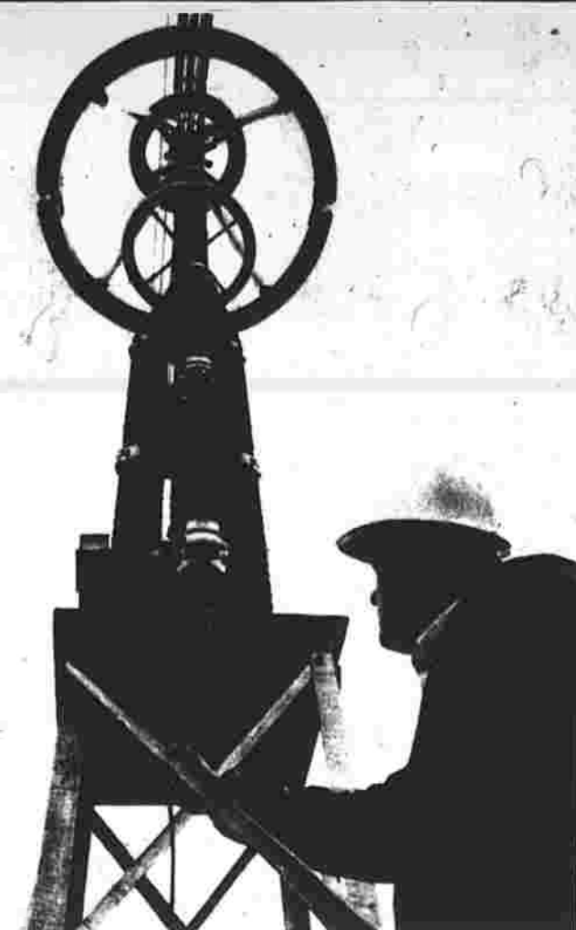
Built to handle blasts of electricity from lightning strikes, and to protect transformers and other expensive electric equipment, this 28-foot-high gapless surge arrester is the first of its kind in the world. It was designed by Westinghouse Electric for the Bonneville Power Administration in Oregon. (UPI photo)
